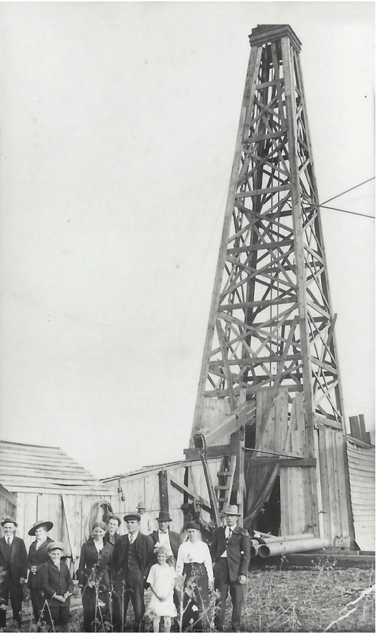
Large quantities of wood were used to build the oil derricks. Each rig included a tall wooden support derrick and the machinery that raised and lowered the drilling equipment. Photo courtesy of Mrs. Homer Honn.
